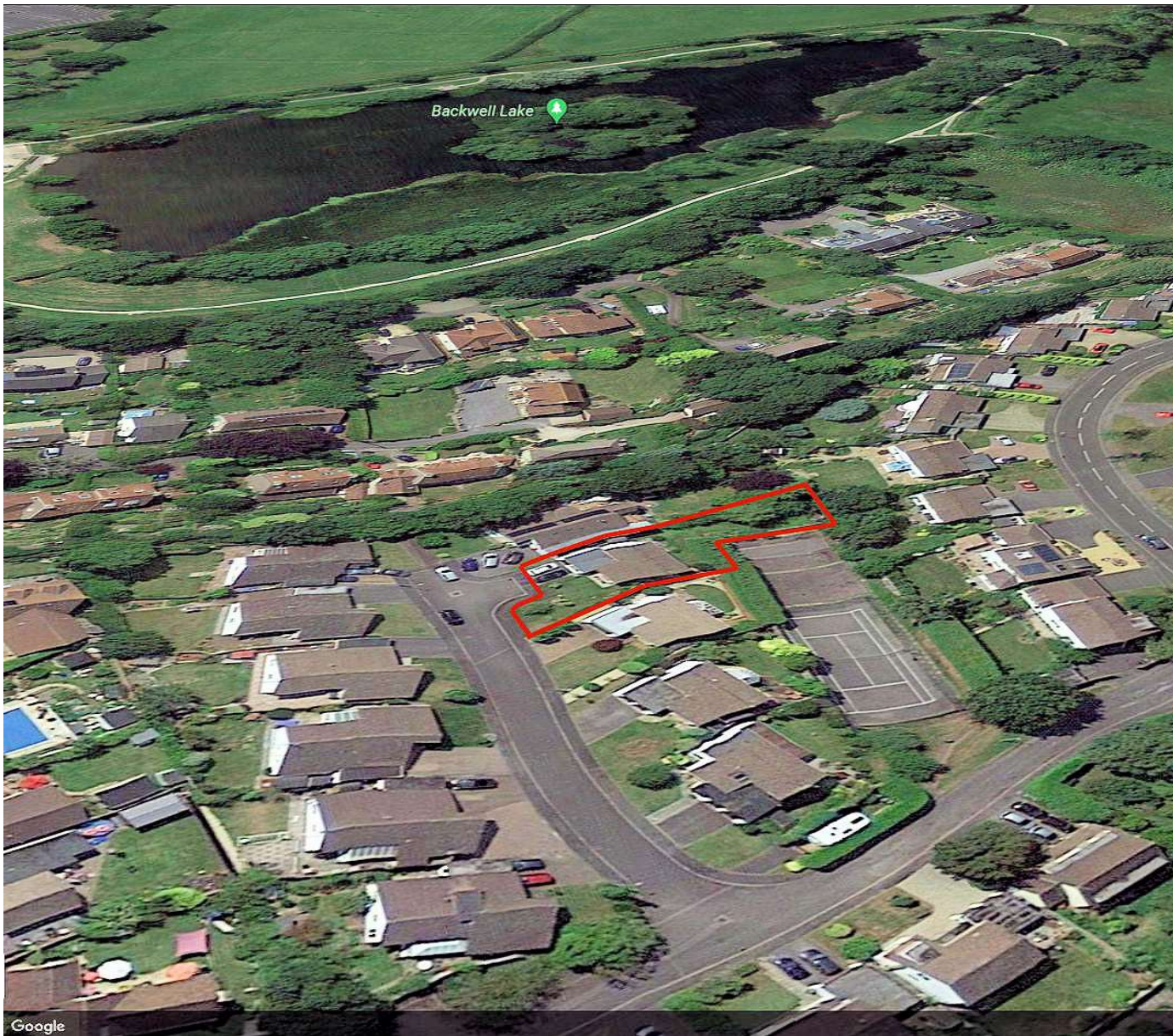
The position in the close facing to the south
